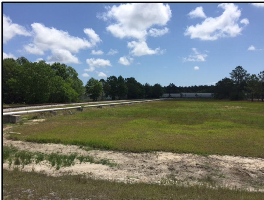
Photograph, facing south, of aboveground pipeline observed on property
