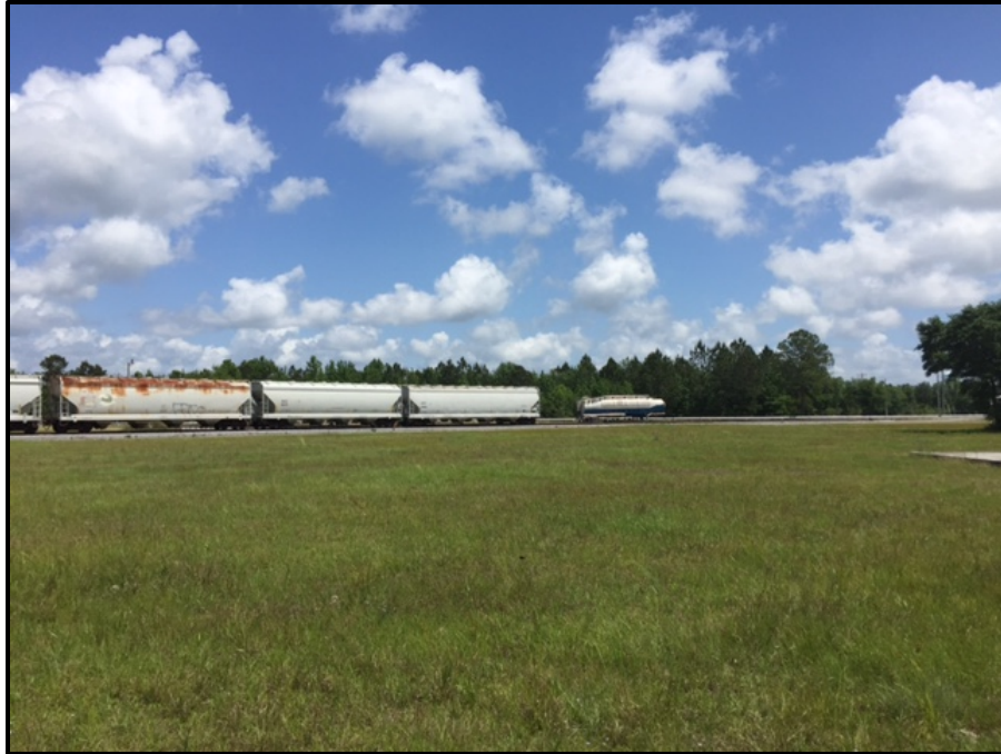
Railroad and dormant rail cars stored on property. Photograph facing southeast.
