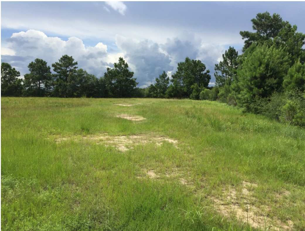
Figure 5. Northwest corner of Site 4, cleared and leveled with signs of canal erosion.
