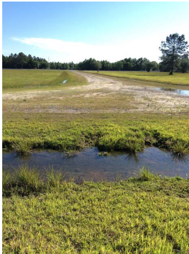
Figure 3. Bermed gravel access roads and drainage ditches in southeastern portion of Site 4.
