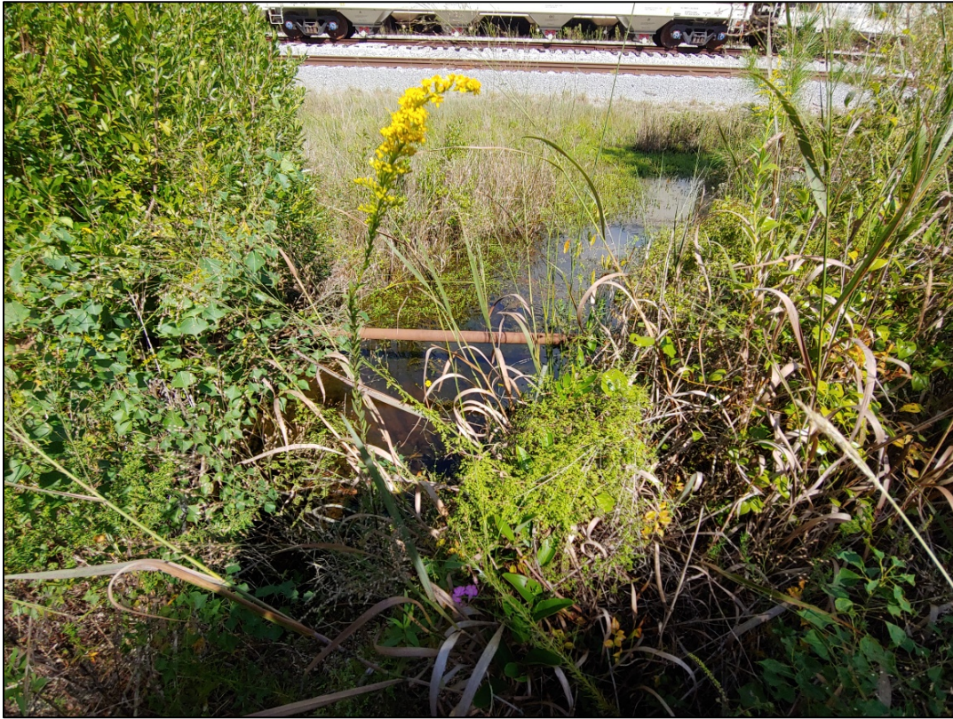
9. Pipeline located in rail spur that splits the Seven States property.
