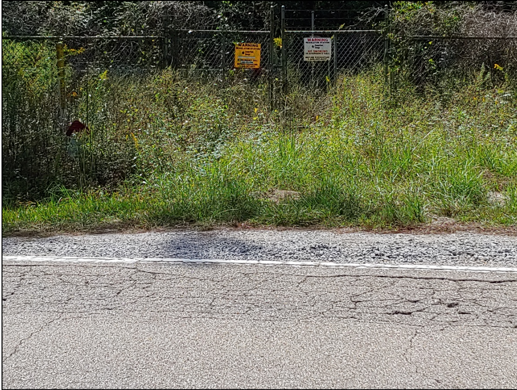
19. Natural gas regulator station, located across Lower Bay Road from the Seven States southern property boundary.
