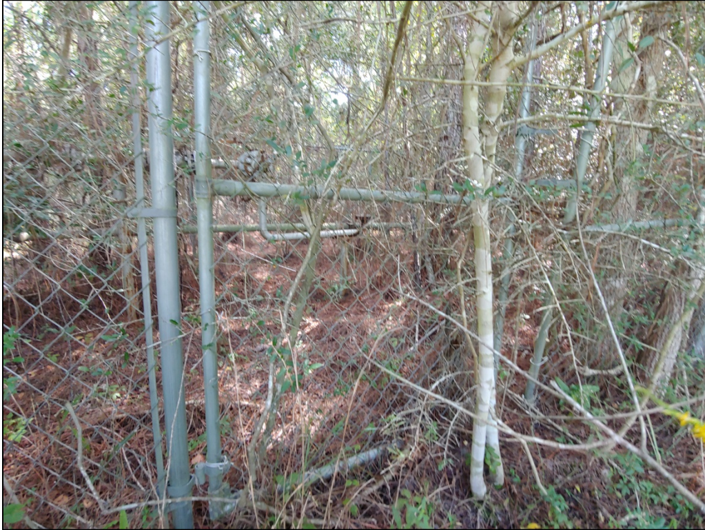
7. Abandoned natural gas well or regulator on south-central portion of Seven States property. Field coordinates 30.241707, -89.535344 (decimal degrees). Natural gas liquid odor (propane like) observed in immediate area.
