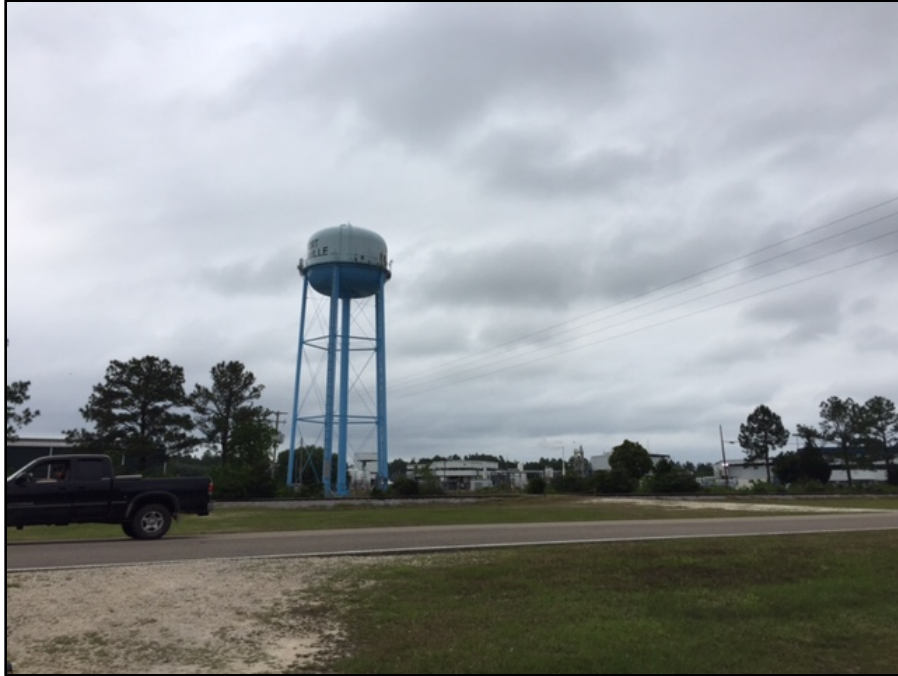
Port and Harbor Drive, across from which is western adjacent water tower. Photograph facing northwest
