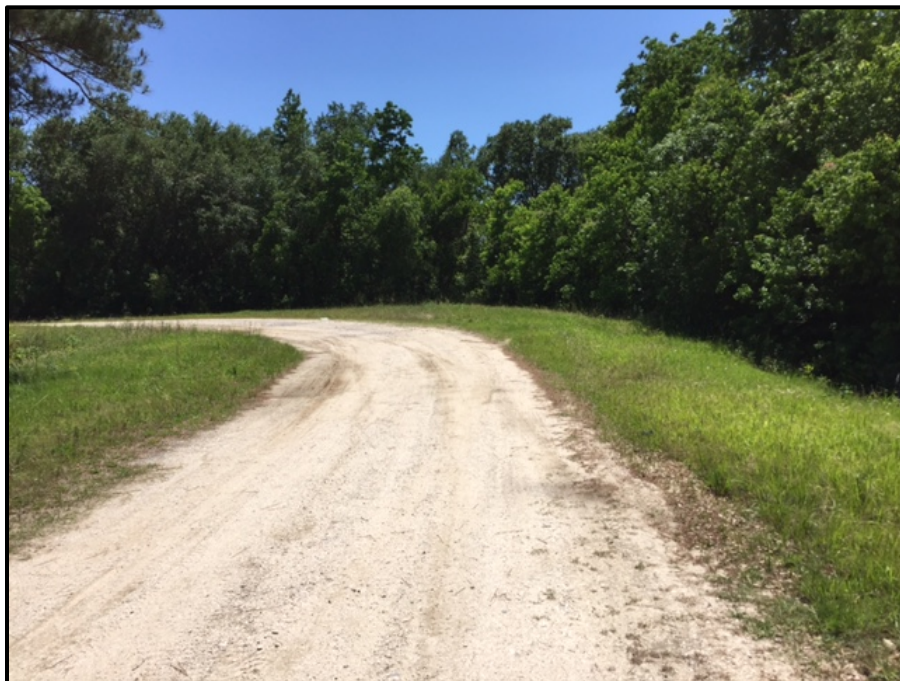
Gravel access road on northern portion of the property , photograph facing west
