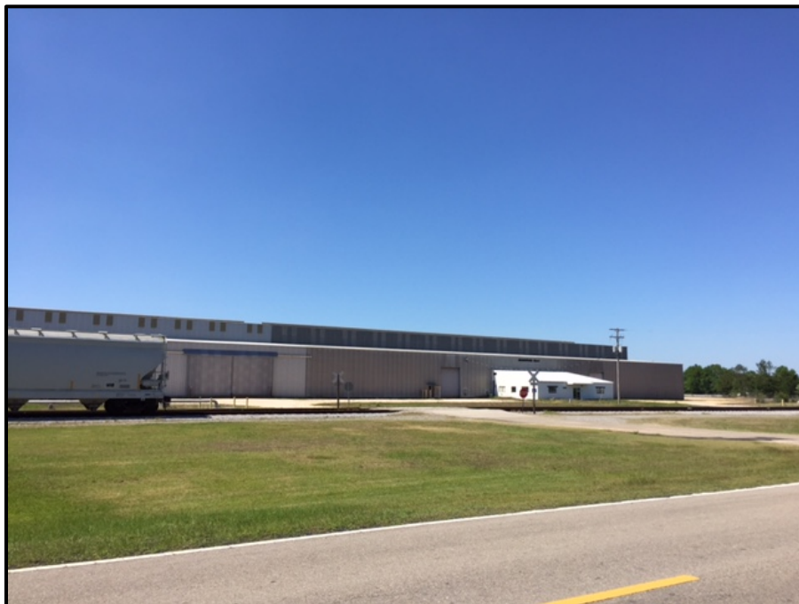
Buildings associated with Port Bienville Port, adjacent to the south of the property
