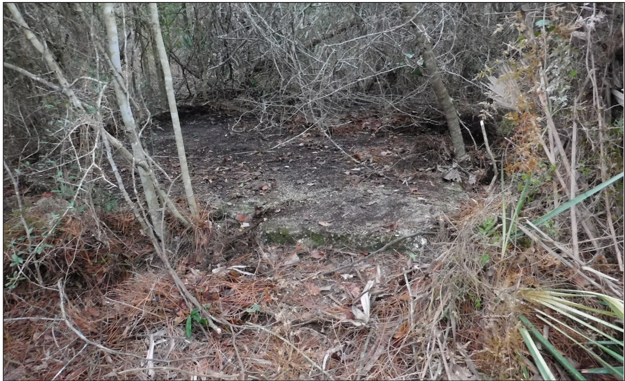
Figure 29. View of concrete slab once cleared at FS-1, facing northeast.
